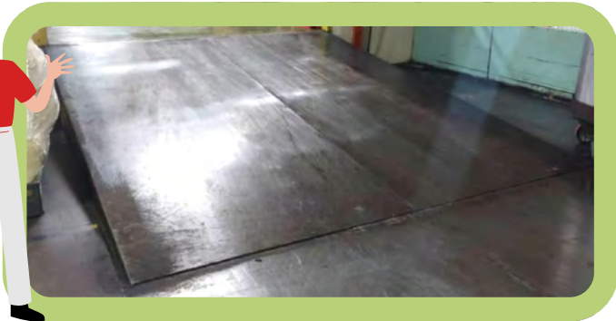
Using a slope to transfer materials
